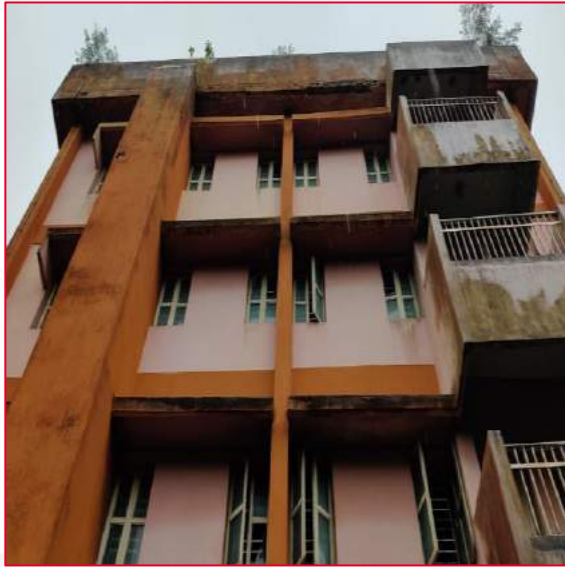
Existing Staff Quarters
