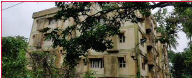
Existing Staff Quarters
